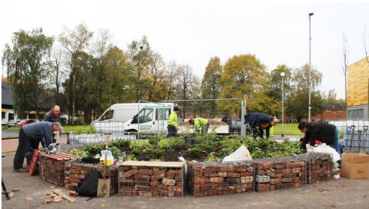
Harpurhey Eco Streets Project (reproduced with permission from Groundwork)
